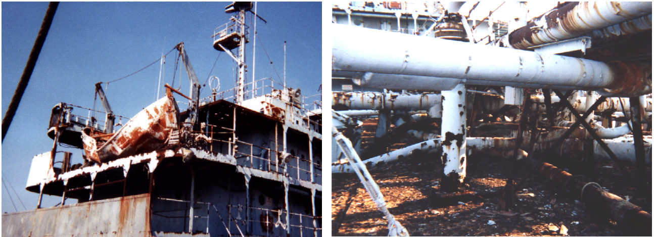
Figure 15. Vessel Deterioration at Beaumont Reserve Fleet
